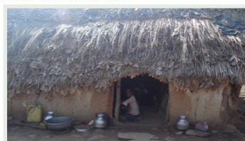
Poor Housing conditions
